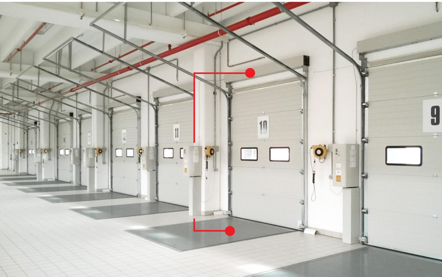
**THE SECTIONAL OVERHEAD DOOR IS A KNOWN ELEMENT** and its characteristics for Loading Bays for dry goods is standardized: insulated 40 mm thick panels one metre high for vertical installations or 610 mm for the others, light RAL 9002 colour, for avoiding heat accumulation, one sight view for outside control or more windows for the light.
