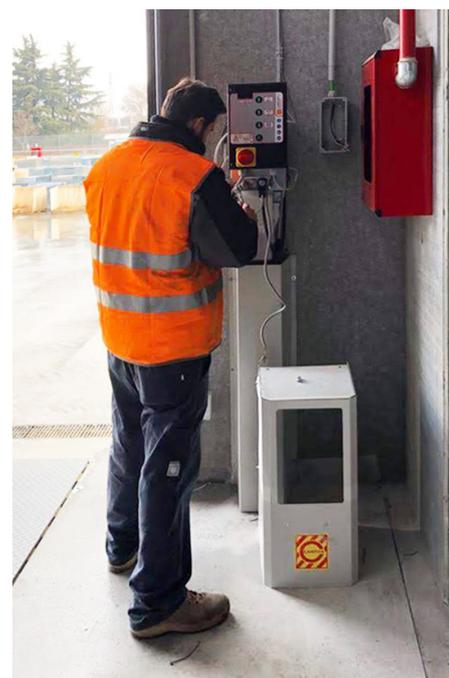
The routine inspection is reduced to the simple oil level check inside the wall positioned CONSOLLE at about 1,5 m H from ground.
